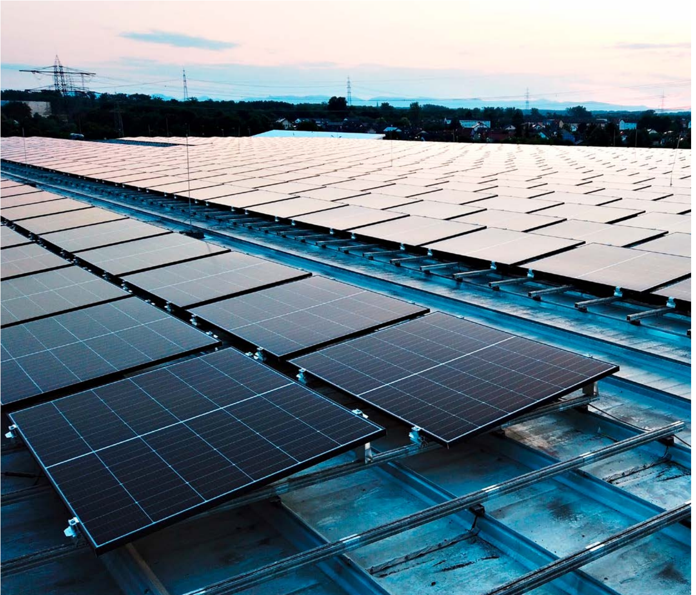
The new modules are mounted at a ten-degree angle and face south.
