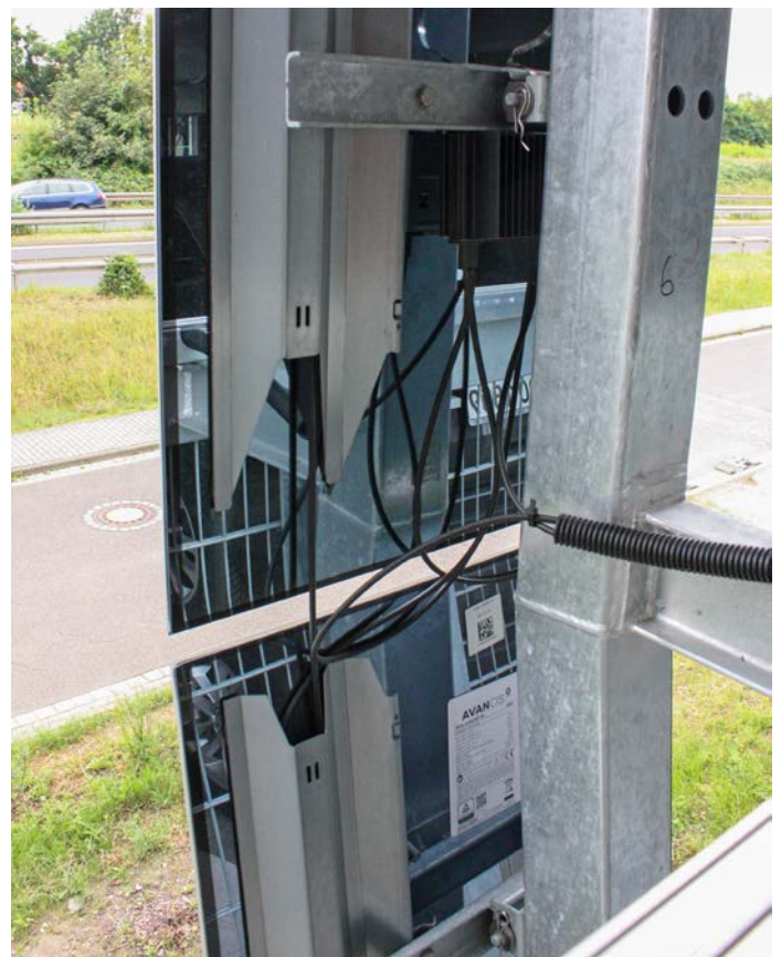
The cables of the modules are fixed to the beams.
