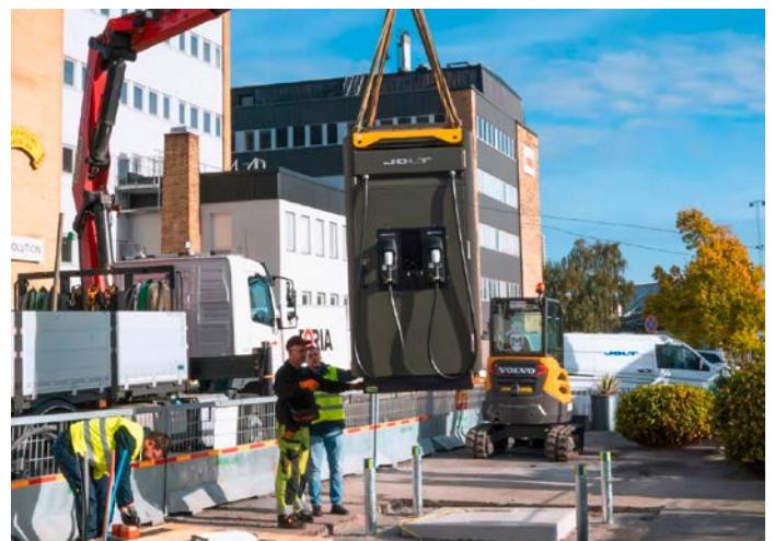
Installation of the fast-charging stations, that are connected to the low-voltage grid.
